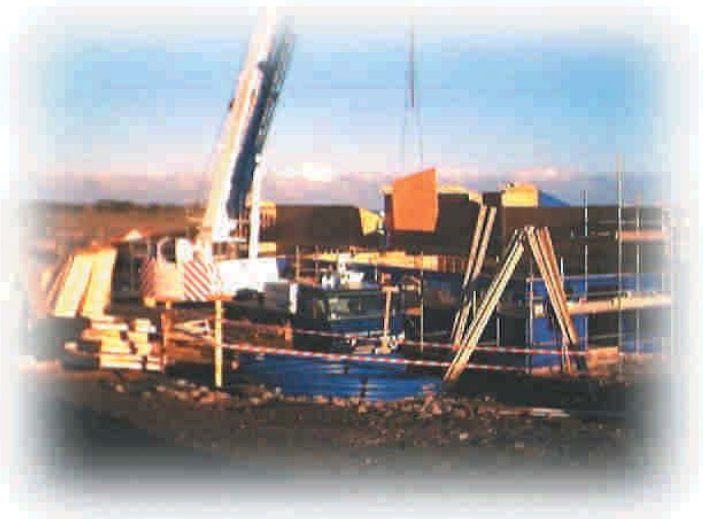
The start of works at Dubford, Aberdeen, for ARK Services Ltd.
