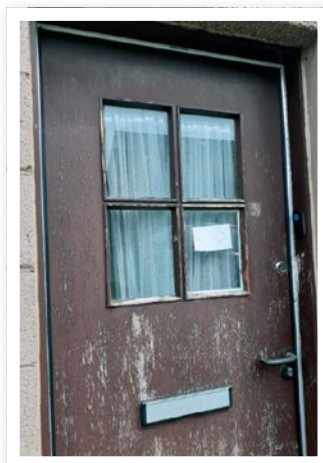
Example of Oxgangs doors before and after.
